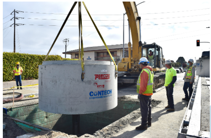
Franklin Storm Drain Extension Project
