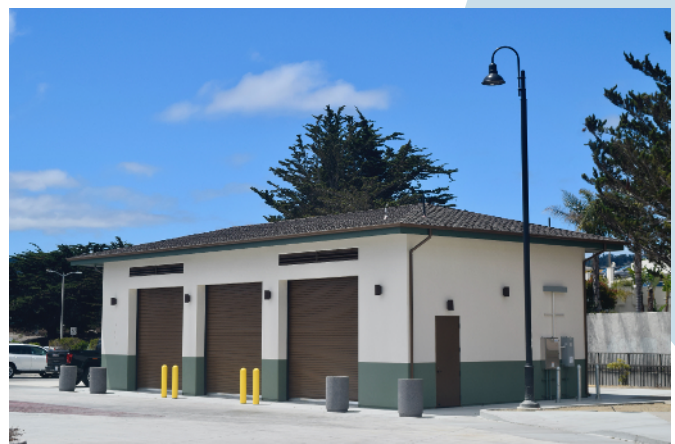
Wharf Trash Compactor Project
